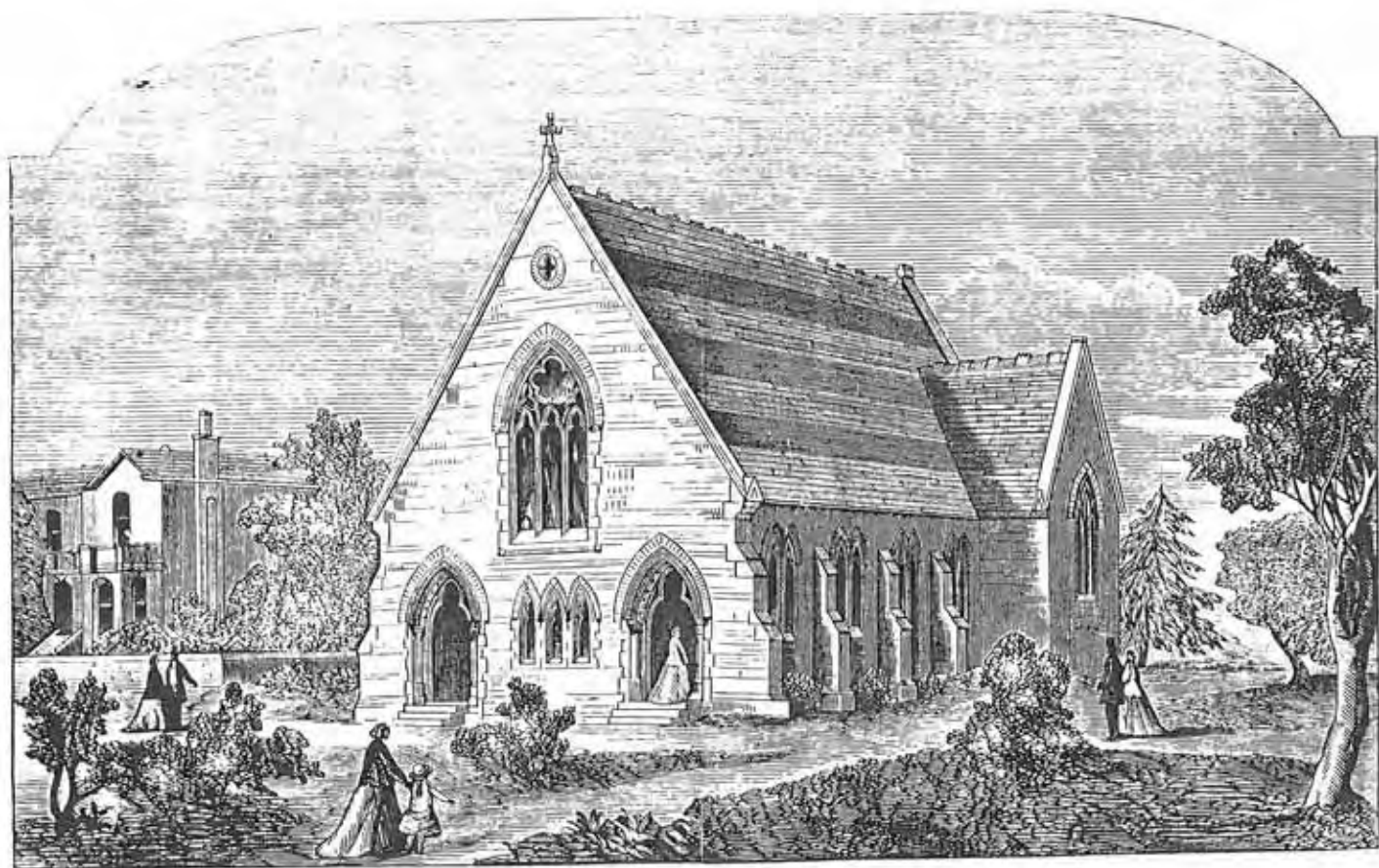
Unitarian Church, Portland Street, SOUTHPORT (Lancashire).
