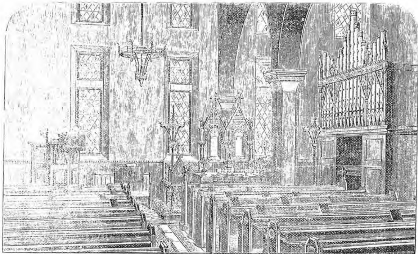
Interior of the Old Meeting House, MANSFIELD (Nottinghamshire).
