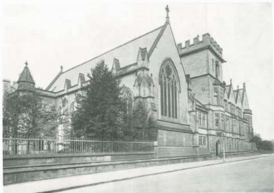
MANCHESTER COLLEGE, OXFORD From the South-East. The Chapel in the Foreground
