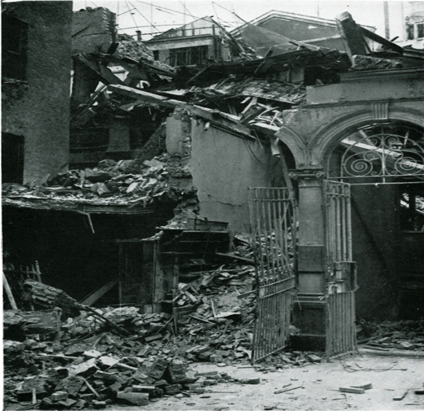
ESSEX HALL ENTRANCE, AUGUST 1944 (WRECKAGE PARTLY CLEARED)
