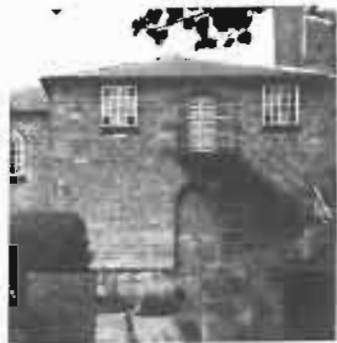
Exterior of Belper.
