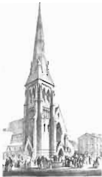
Above: Hope Street, Liverpool. Built for Martineau in 1849, demolished 1963.
