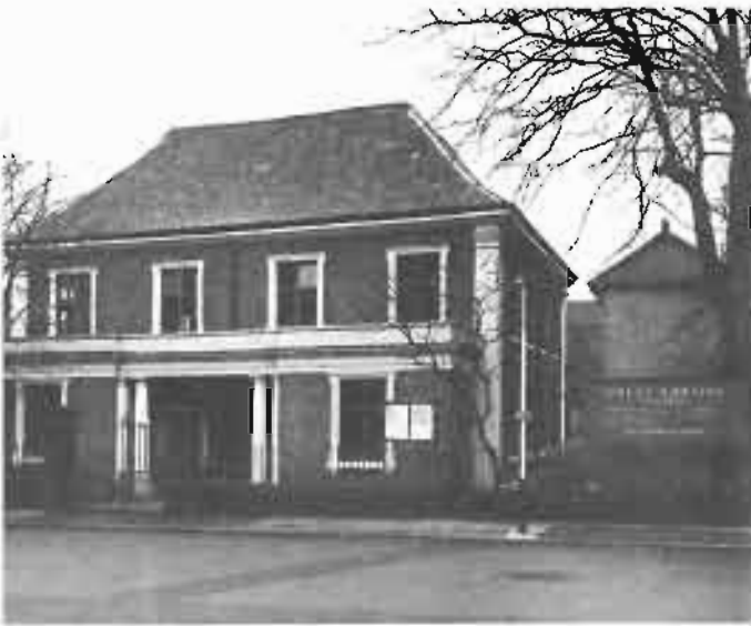
Left: Great Meeting, Leicester (1708). Probably the first brick building in Leicester. Right: part of Hinckley Unitarian Chapel showing brick pilasters (1722).
