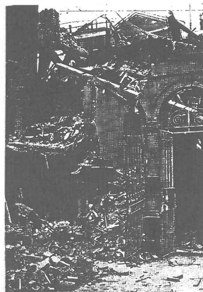
ESSEX HALL ENTRANCE, AUGUST 1944 (WRECKAGE PARTLY CLEARED)
