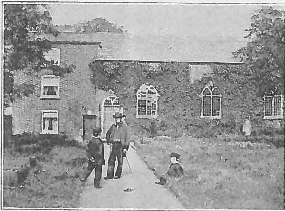
OLD CHAPEL, DOB LANE, FAILSWORTH
